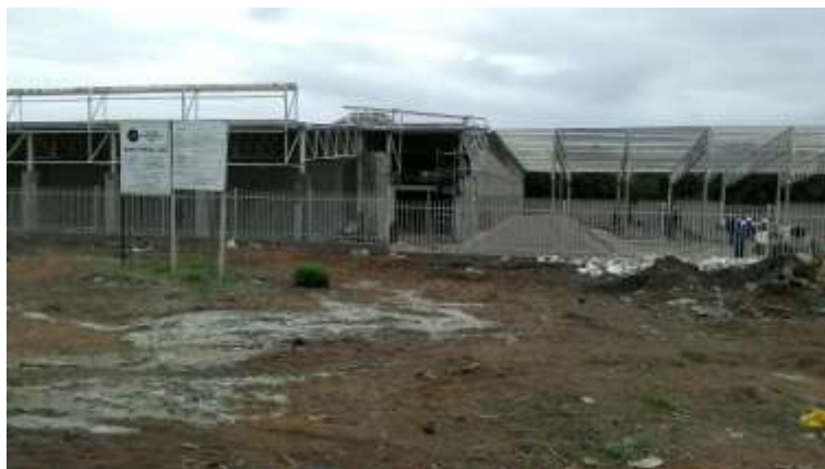
Shoprite construction site, Maputo
