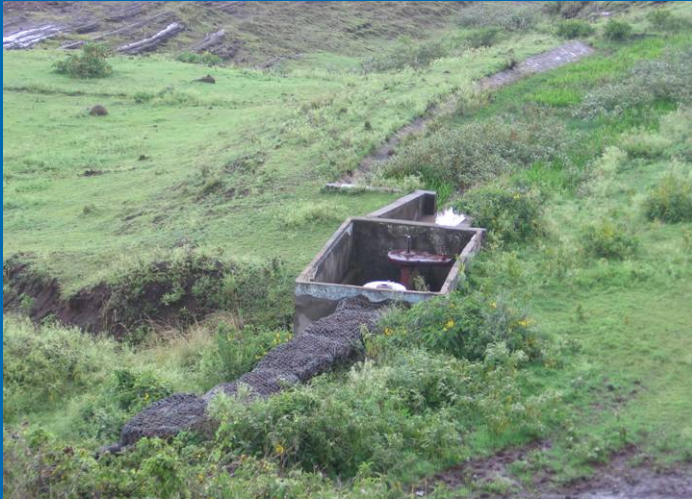
Main regulatory gate of Belbela dam
