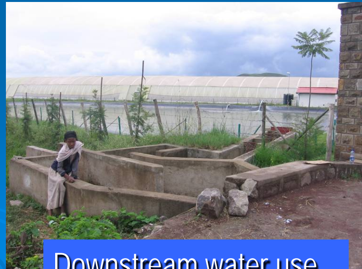
From Belbela to Filtinno Division Box: 9 small gates for farmers' fields
